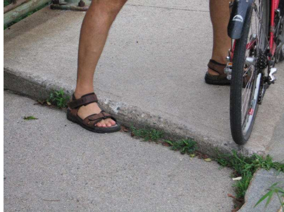
Figure 4 Transition Over Railroad Bridge east of BU Bridge
